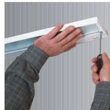
Step 3 Mount fixture to cabinet bottom using captive mounting screws.
